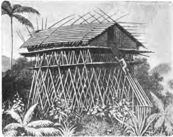
FIG. 15.—The Arfaks of New Guinea make their houses as all others have done, but secure protection from enemies by mounting them on poles high in the air.
